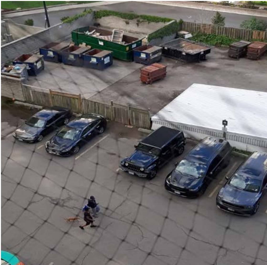
Figure 13: Outdoor waste enclosure at a private rental building in St. James Town. There are no black bins for garbage.
