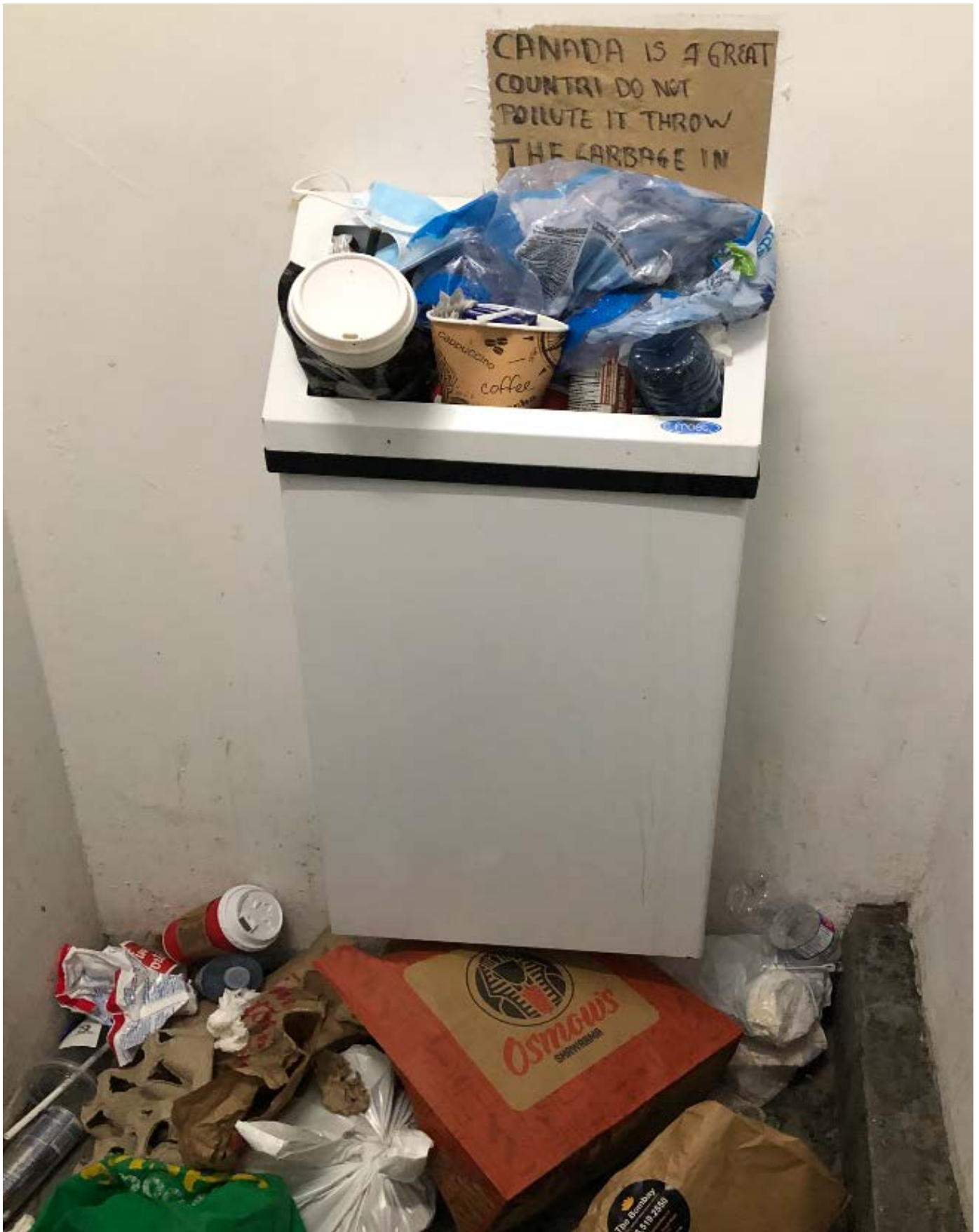
Figure 4: Basement waste receptacle in Building X, a private rental building in St. James Town.
